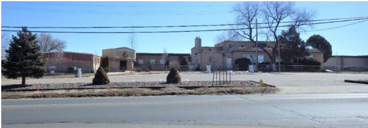
Photo 4. Current Road Conditions in Front 5AM.3975—Irondale School, view to east.
