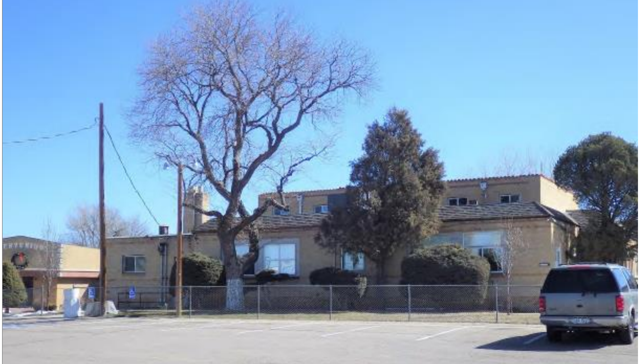
Photo 3. 5AM.3975—Irondale School, view to east.
