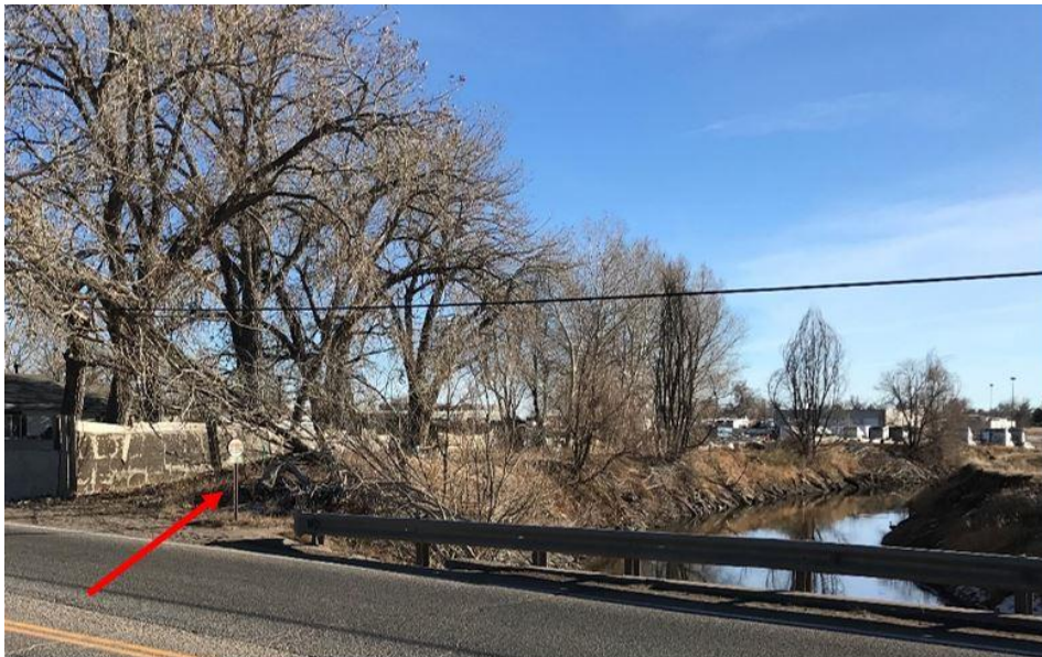
Photo 22. 5AM.477—O'Brian Canal. View south from E. 88th Avenue bridge looking at closed ditch rider road with modern berm blocking entry on east side of canal, view to south
