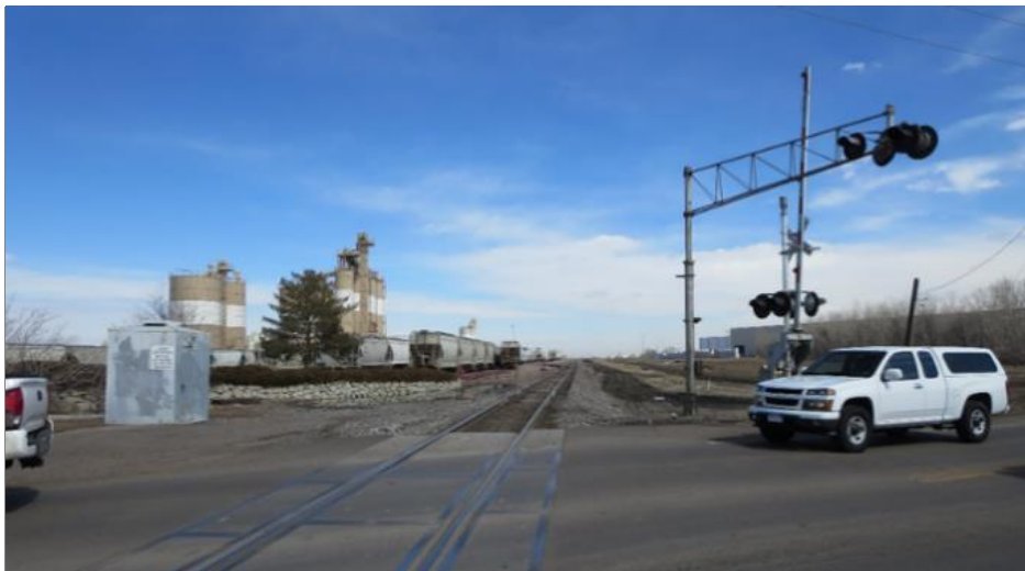
Photo 14. 5AM.459—Denver Pacific/Union Pacific Railroad. At the intersection of E. 88th Avenue; view northeast
