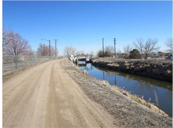
Photo 18. 5AM.477—O’Brian Canal north of E. 88 th Avenue, view to the north,
