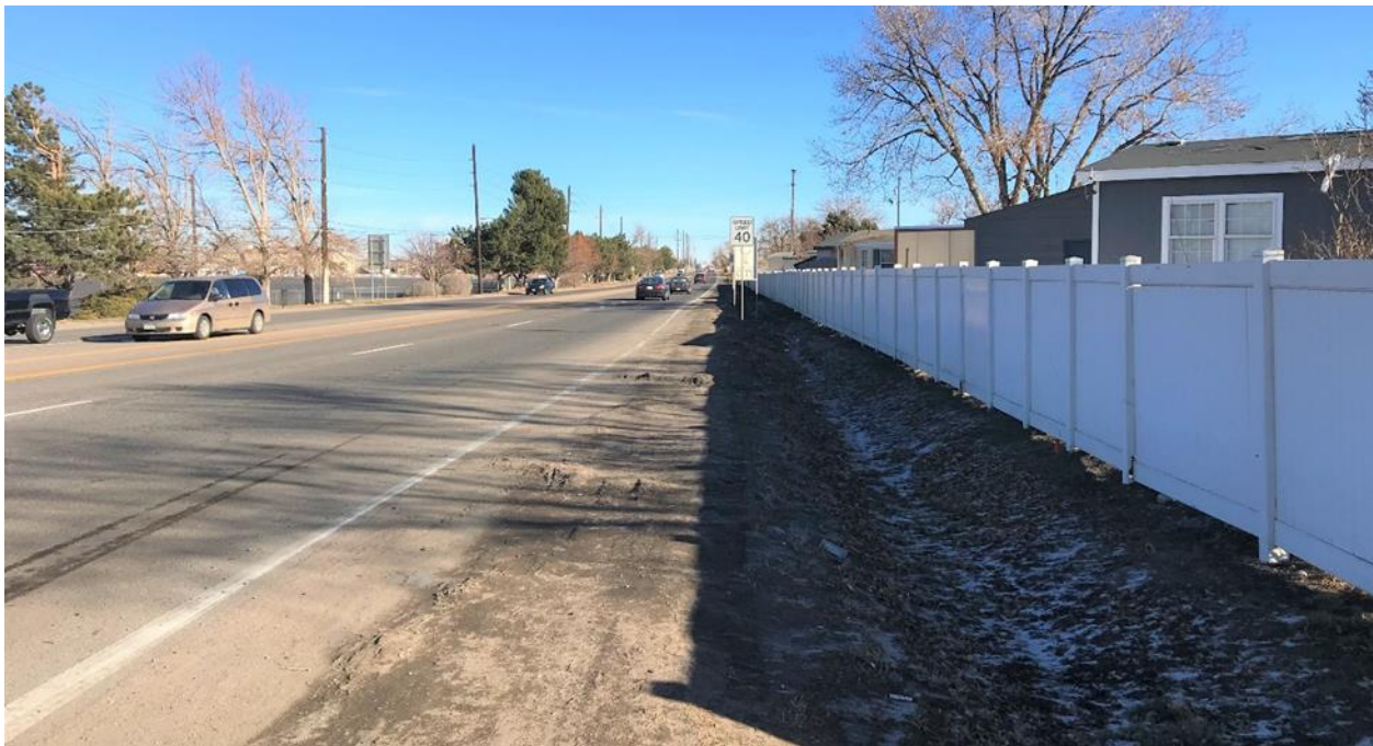
Photo 11. 5AM.3990—Wikiup Mobile Home Park. View to east on 88th Avenue from Wikiup entrance. Existing non-historic vinyl fence shown on right; new noise wall to be built on north (left) side of vinyl fence and drainage ditch.
