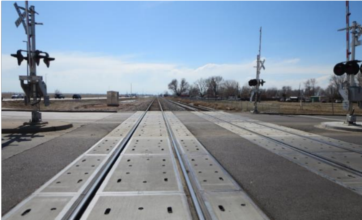
Photo 15. 5AM.464—BNSF railroad tracks. At 88th Avenue crossing, view southwest
