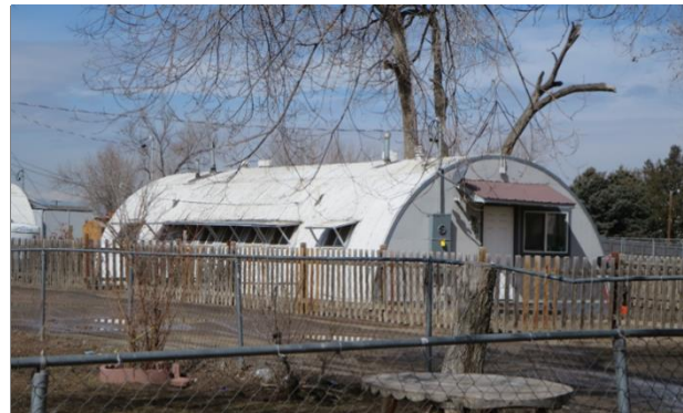
Photo 12. 5AM.3994—Country Cottages Quonset Park, view to west.
