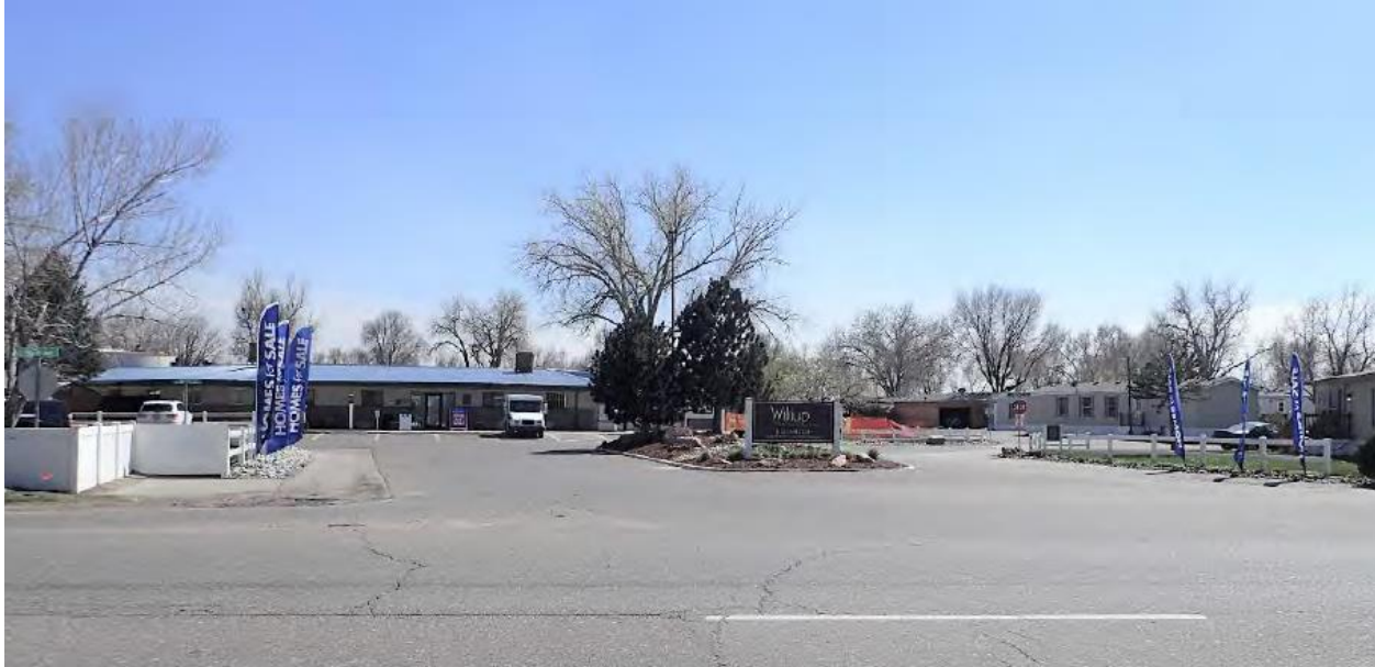
Photo 10. 5AM.3990—Wikiup Mobile Home Park. View to south from 88th Avenue towards Wikiup entrance.
