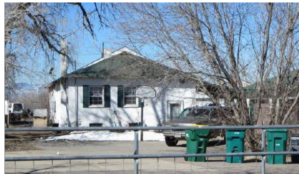
Photo 5. 5AM.3976—8705 Rosemary Street, view to west.
