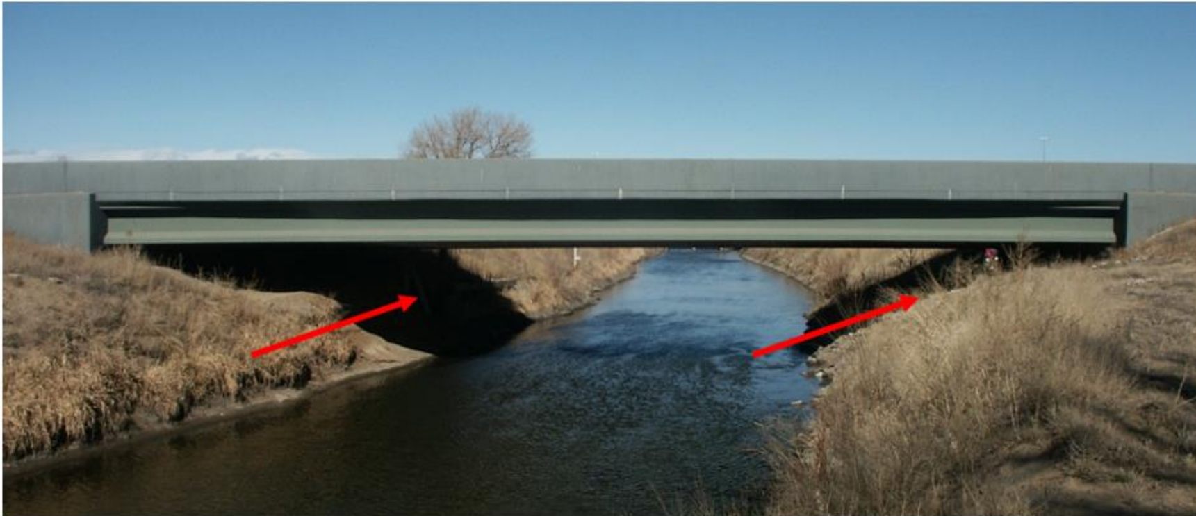
Figure 31. Crossing of Sable Boulevard with O'Brian Canal. The bridge is located approximately 5.3 miles northeast of e. 88th avenue. The proposed bridge at E. 88th avenue will be of similar bridge type and appearance, with sloped geometry under the bridge (red arrows). View southeast. Photo Courtesy: CDOT.
