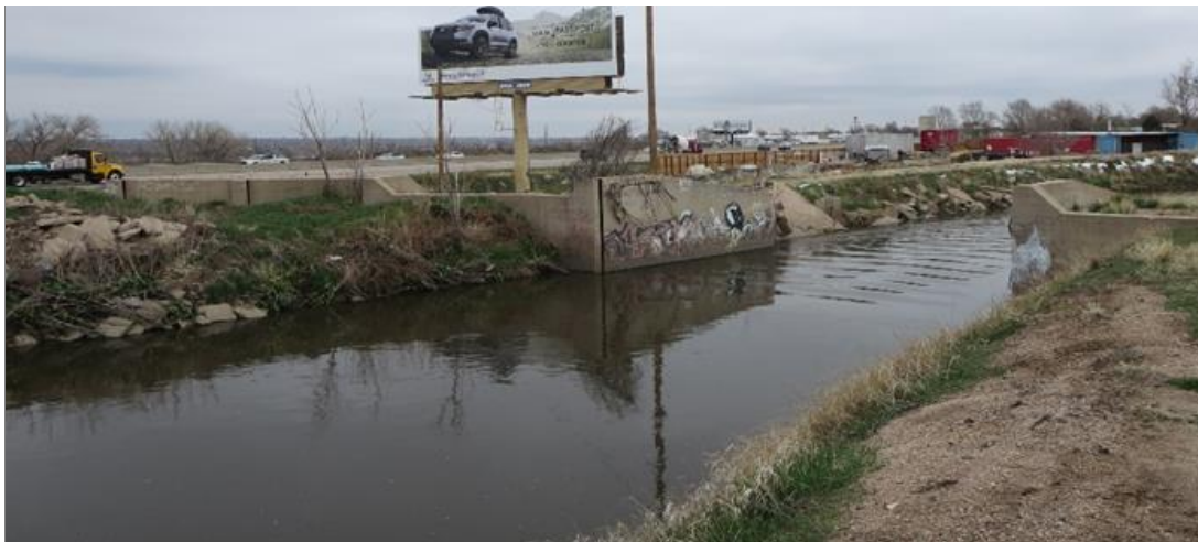
Photo 16. 5AM.465—Burlington Ditch, view at decommissioned bifurcation gate.
