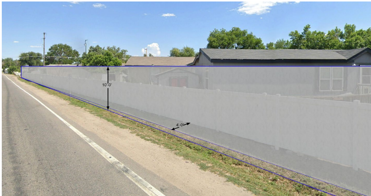
Figure 14. Recommended Noise Barrier at Wikiup Community
