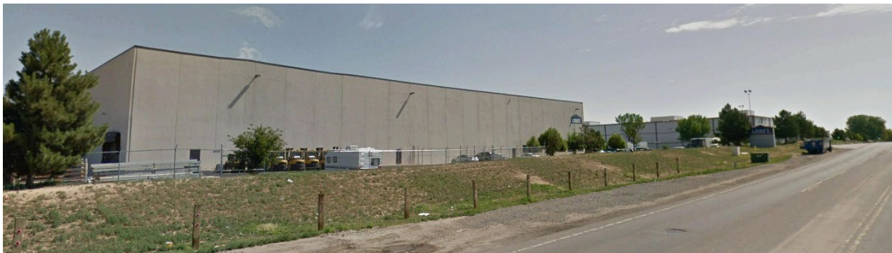
Photo 4. Industrial Land Use (Medium) (Looking northeast from E. 88th Avenue, east of Rosemary Street)
