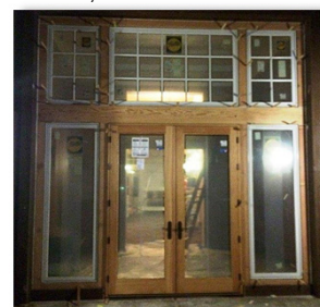
New entry door
